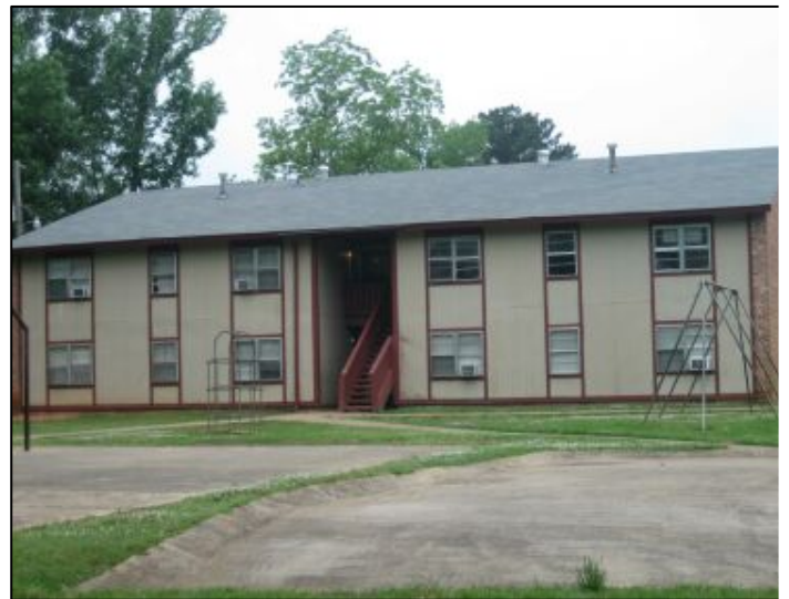
Photo: Union Square Apartments Exterior Backside – Before Rehab
