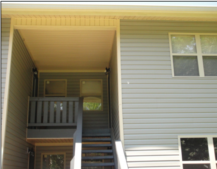
Photo: Close up - New Exterior Stairs, Vinyl Siding, and Energy-Efficient Double-Pane Windows
