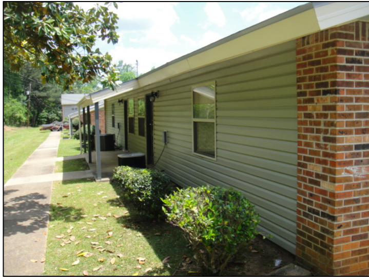
Photo: One Bedroom Senior Building (Frontside) - New Vinyl Siding and Energy-Efficient Double-Pane Windows
