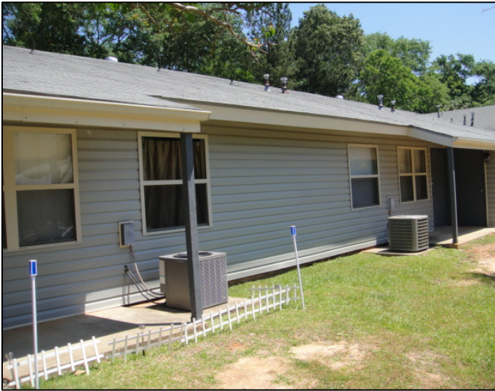
Photo: One Bedroom Senior Building (Backside) - New Vinyl Siding and Energy-Efficient Double-Pane Windows
