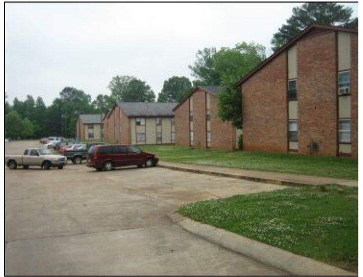
Photo: Union Square Apartments Exterior (curbside) – Before Rehab
