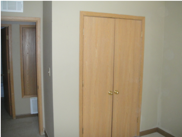
Photo: New Interior Closet Doors to replace old Bi-fold Doors that were falling off the track.
