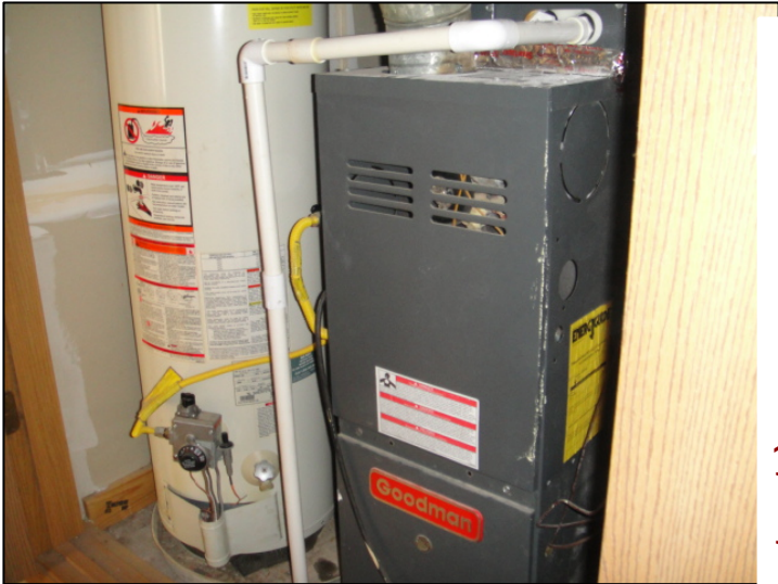
Photo: New Hot Water Heaters and Furnaces
