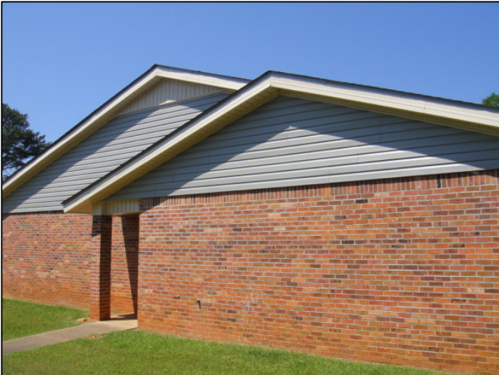
Photo: One Bedroom Senior Building (Side) – New Vinyl Siding
