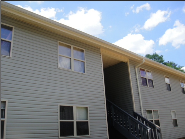
Photo: New Vinyl Siding and Energy-Efficient Double-Pane Windows
