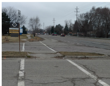
Curbed island at Walli Strasse Drive
