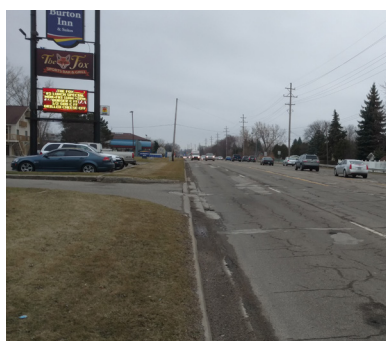
North end of the project
