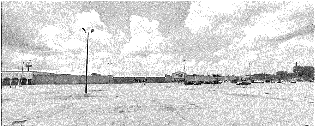
Figure 3. Current Facade and Condition of Building.
