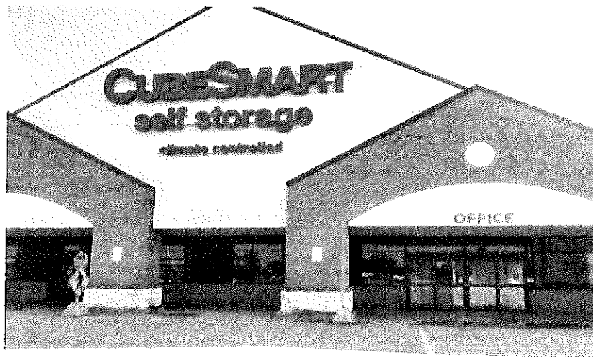
Figure 2. Repurposed Indoor Storage Building in Southgate, Michigan.
