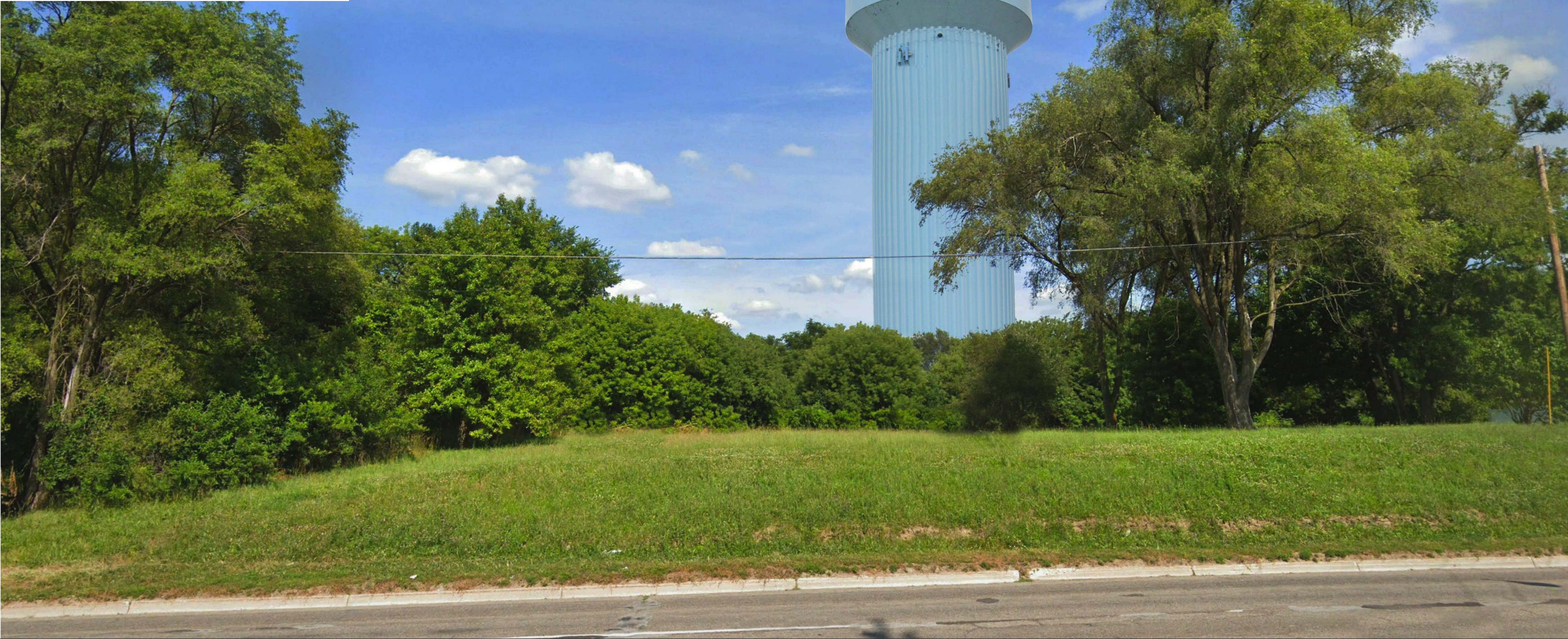
BURTON ELEVATED WATER STORAGE TANK | EASTERN PERSPECTIVE | 3063 SOUTH CENTER ROAD PERSPECTIVE | BURTON, MICHIGAN | JUNE 2020
